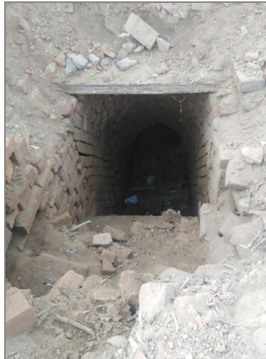
Figure 25-26: Underground room has blocked due to rain (Source: Author)
