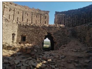
Figure 27-29: Bricks used in the fort's erection currently lie at the bottom of its damaged and cracked outer walls (Source: Author)
