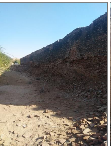
Figure 30-32: Bricks used in the fort's erection currently lie at the bottom of its damaged and cracked outer and inner walls (Source: Author)
