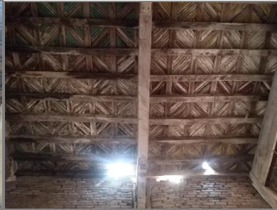
Figure 16: Traditional tarseem bandi technique at the ceiling of the fort's room (Source: Author)
