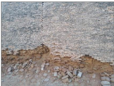
Figure 27-29: Bricks used in the fort's erection currently lie at the bottom of its damaged and cracked outer walls (Source: Author)
