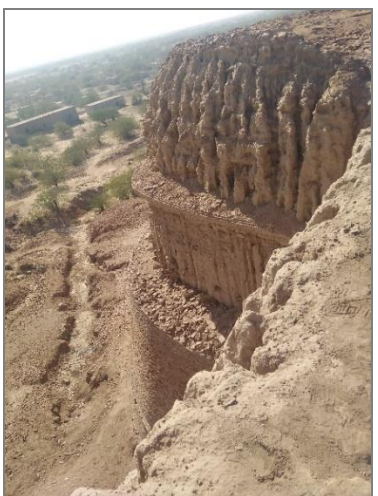
Figure 30-32: Bricks used in the fort's erection currently lie at the bottom of its damaged and cracked outer and inner walls (Source: Author)
