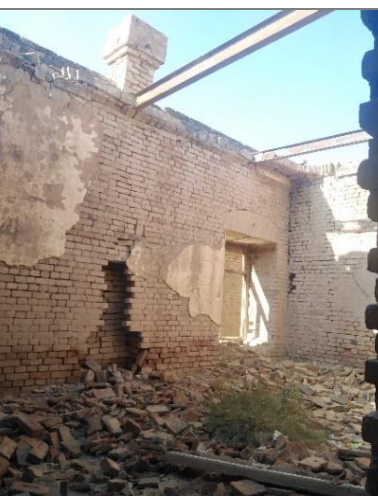
Figure 30-32: Bricks used in the fort's erection currently lie at the bottom of its damaged and cracked outer and inner walls (Source: Author)
