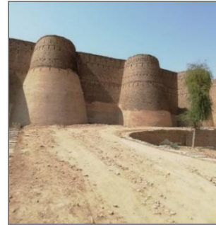
Figure 38: 62-foot deep bastion of the Derawar Fort has been repaired up to a height of 75 feet (Source: Author)
