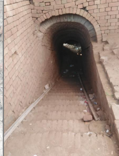
Figure 25-26: Underground room has blocked due to rain (Source: Author)
